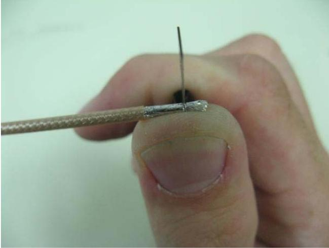
14) Use the plier to break off the tinned tip, exposing the center.
