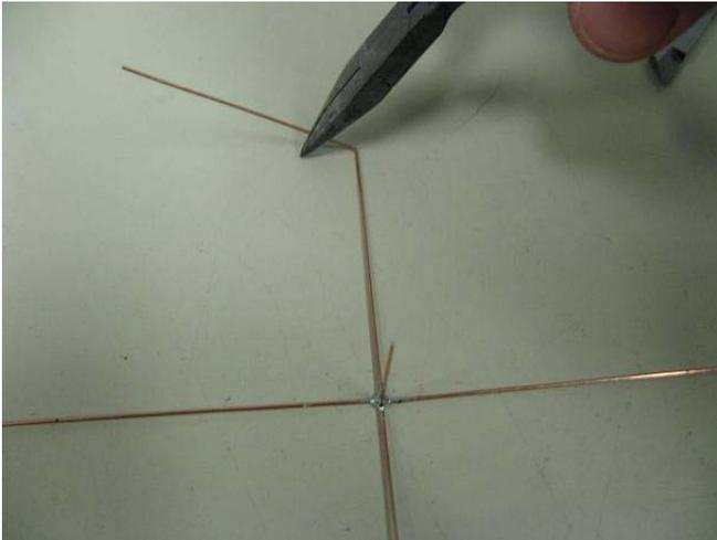
11) Hold the arms with plier and adjust angle to 45deg. by twisting the ends. To get 45deg, the whole thing should lay evenly on its five legs. This way, pitch angle is exactly 45deg.
